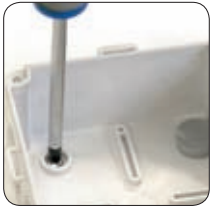
Fix the box and cover the screws with the caps.
