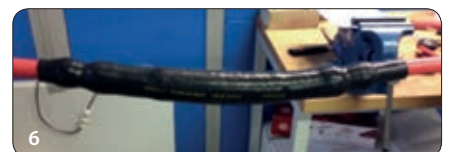
6 The joint is ready and can be used immediately
