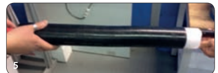
5 The outer protective sheath is positioned and installed
