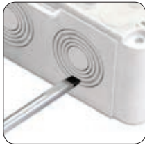
Knock out the pre prepared holes.
