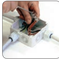
Insert the cables and connect the wires.
