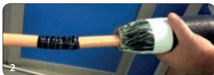
2 The joint is fitted on the connected cable
