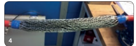
4 The metal shield is rebuilt
