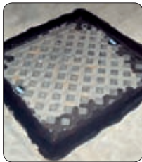
Scellage des cockpits
