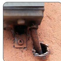
Corrugated pipe entry protection
