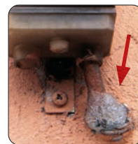
Corrugated pipe entry protection
