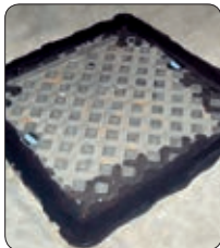
Scellage des cockpits
